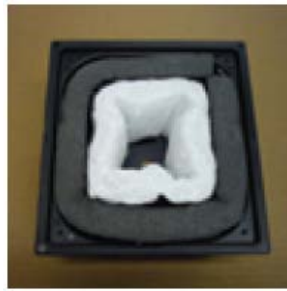
Fig.2 Install 3M foam and acoustic insulation.
